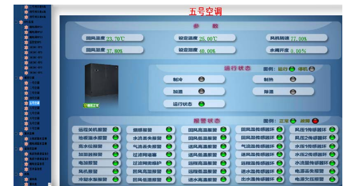
Weibo Server Rooms Parameter Control Panel
